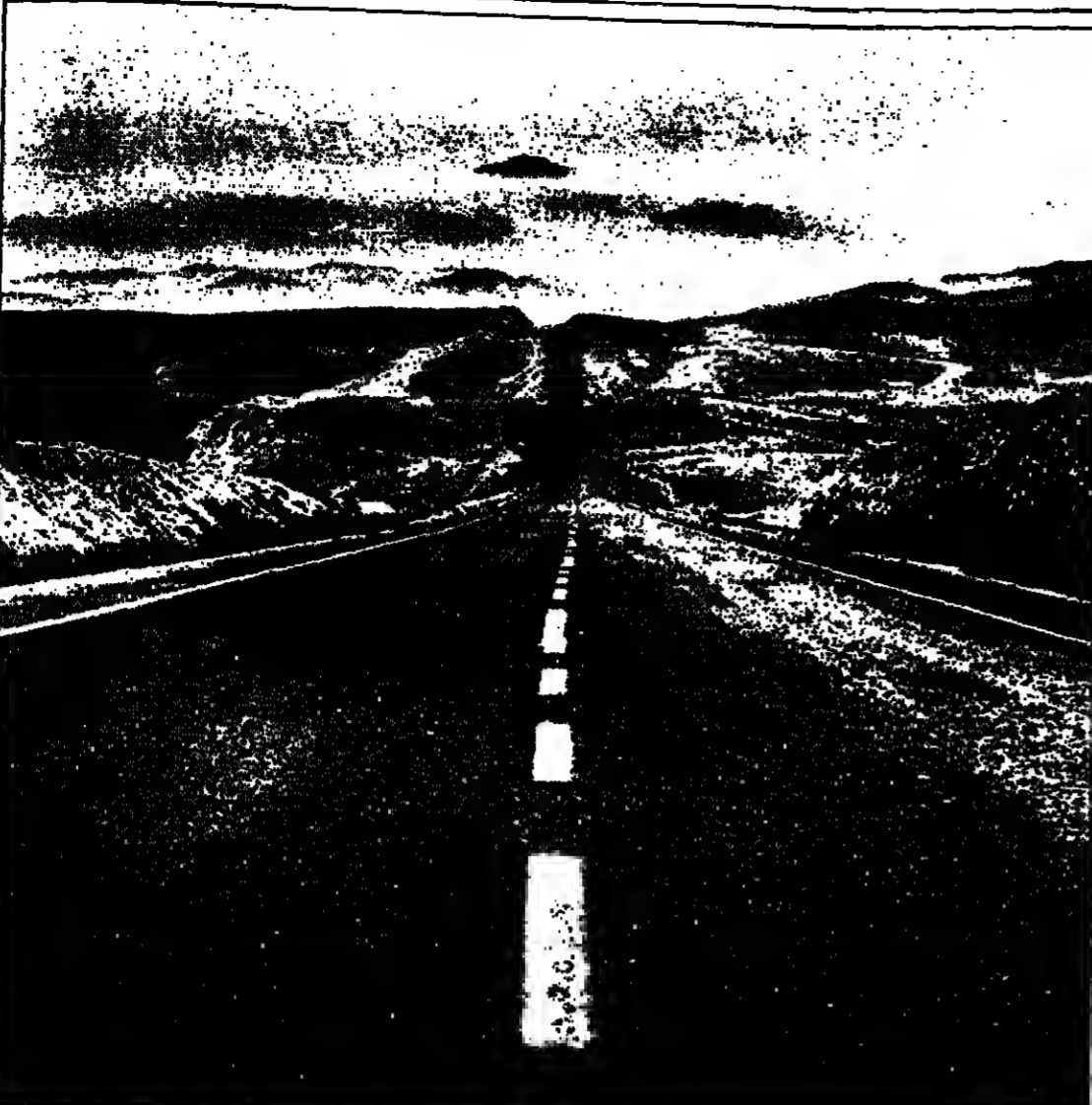
Officials have found that heat, dust and sand, as well as many heavy vehicles on relatively few roads, are the main reasons for erosion of road markings.
